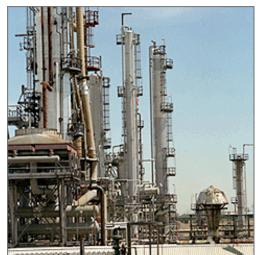
An oil refinery has lots of towers where oil is heated until it turns into a gas that rises. Different types of oil can be separated because they turn into liquid at different temperatures as they cool. Department of Energy.
