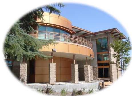
CSUN Police Services is located at the corner of Darby Ave. & Prairie St., just west of the B3 parking structure.
