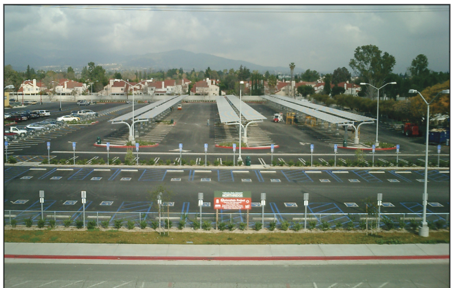
Figure 27. First PV array at California State University, Northridge. Installed in parking lot E6.
