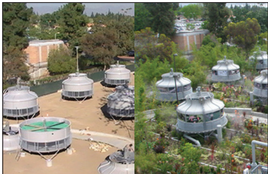
Figure 25: Rain forest during construction, 2007
