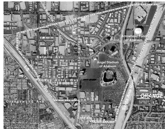
Aerial photograph of the project area.
