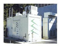
In 2001, CSUN installed six microturbines through a partnership with the South Coast Air Quality District and LADWP as a way to save energy and reduce its reliance on the state's fragile electrical grid.
