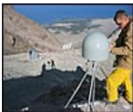
GPS receiver installation
