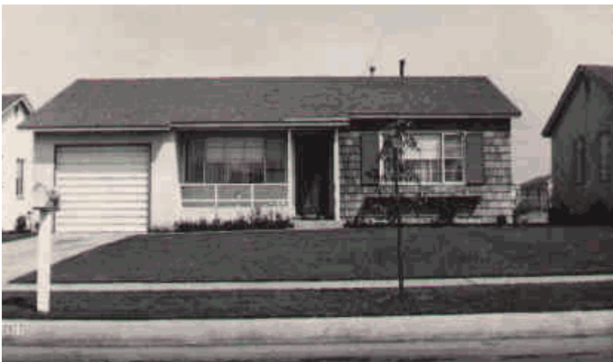
The first house built in Pacoima.
