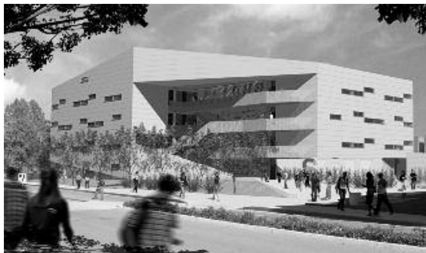
Work has begun on Chaparral Hall, CSUN's new state-of-the-art science building planned for the campus' southeast sector. It is expected to "come on board" in 2009.
