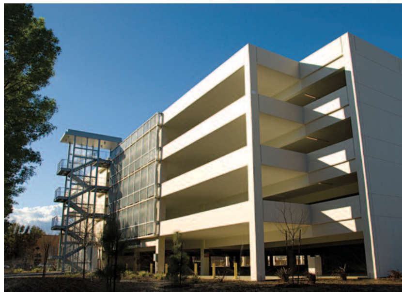
The G3 Parking Structure, off Zelzah Avenue between Prairie and Dearborn streets, opened Jan. 29. The new structure and the surrounding lots add 1,840 new parking spaces to campus, including 118 for faculty and staff and 49 for disabled people.
