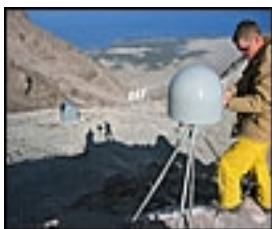
GPS receiver installation
