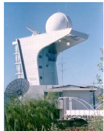
Figure 4: two examples of the telescope domes. (left) Dutch open telescope. This telescope is kept with open enclosure. (Right) Retractable dome at Huairou Solar Station in China. The dome can be moved away from the telescope during good weather conditions.
