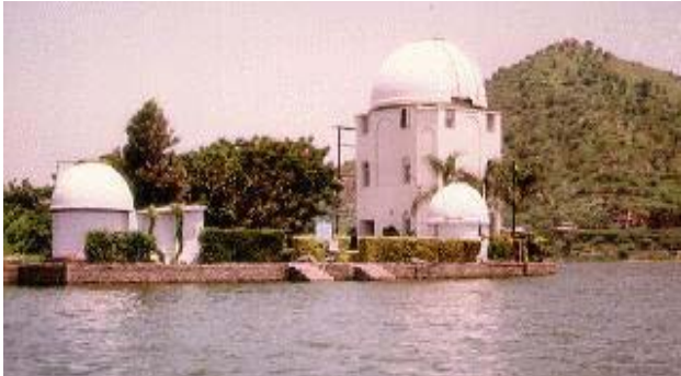
Figure 2: Udaipur solar observatory on an island. (Up) with water body around the lake (down) during the dry conditions.
