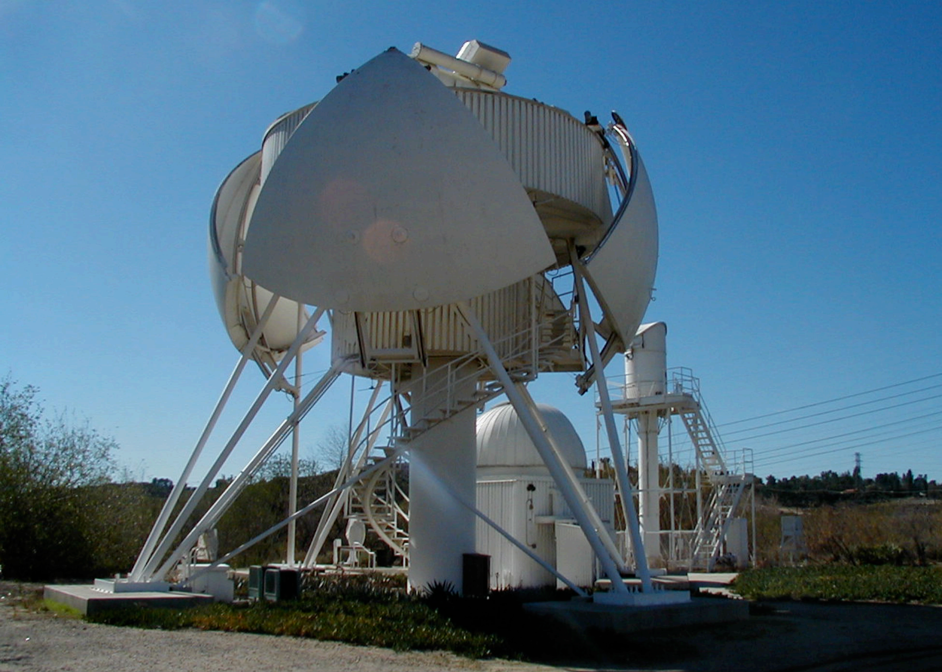
Built in the early 1970's the San Fernando Observatory has extensive ground-based solar irradiance measurements.
